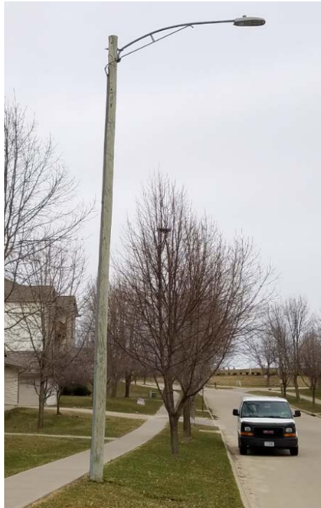
A. Existing Utility Poles
