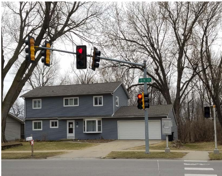
B. Non-Ornamental Municipal Service Pole
